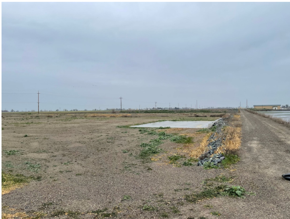
Figure 1-5 City of Colusa Biosolids Drying Area and Stock Piling Surface
