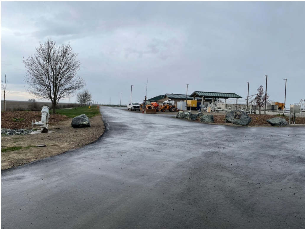
Figure 1-4 City of Colusa WWTP Entrance Landscaping and Grass Planting
