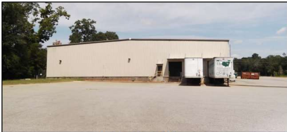
View of Rear of Building
