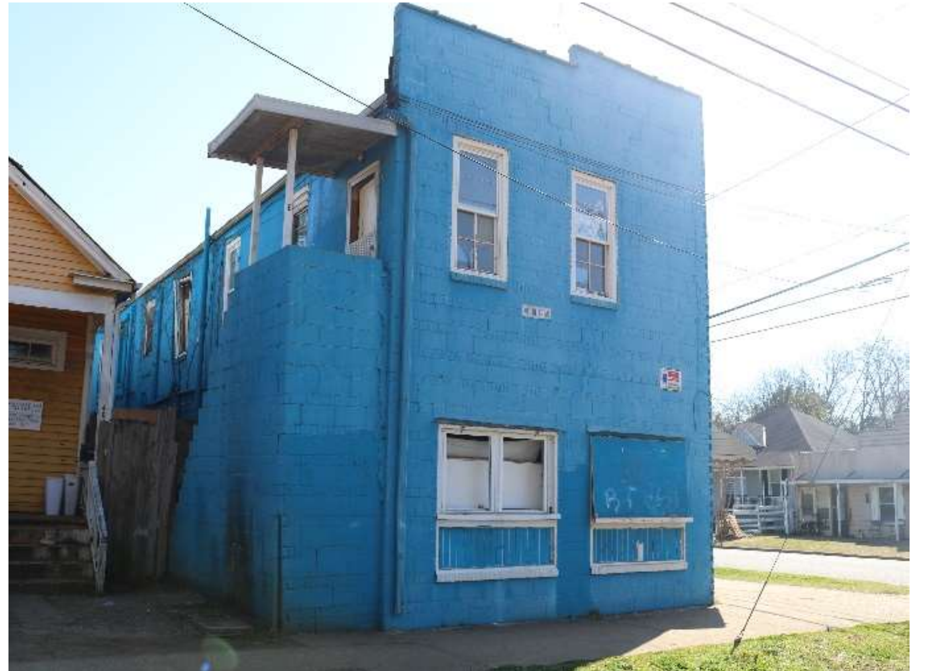
Cozy Corner Pre-Demolition
