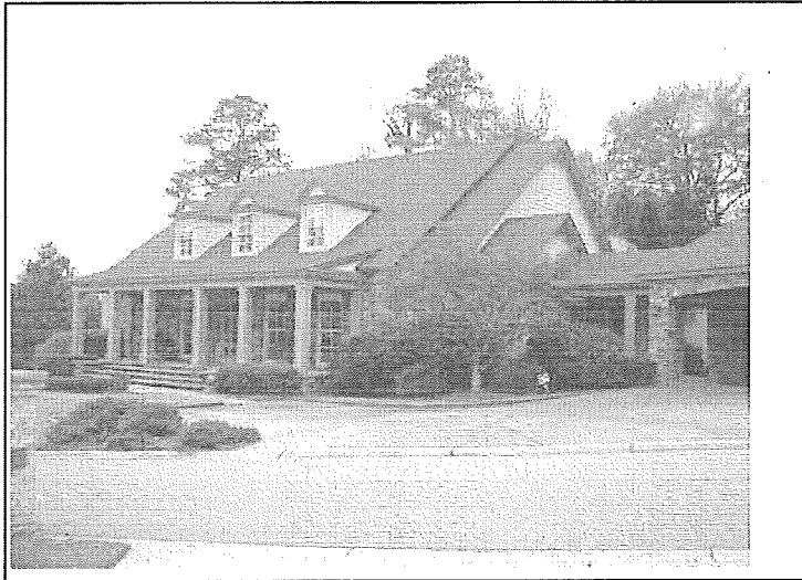
FRONT OF SUBJECT PROPERTY
