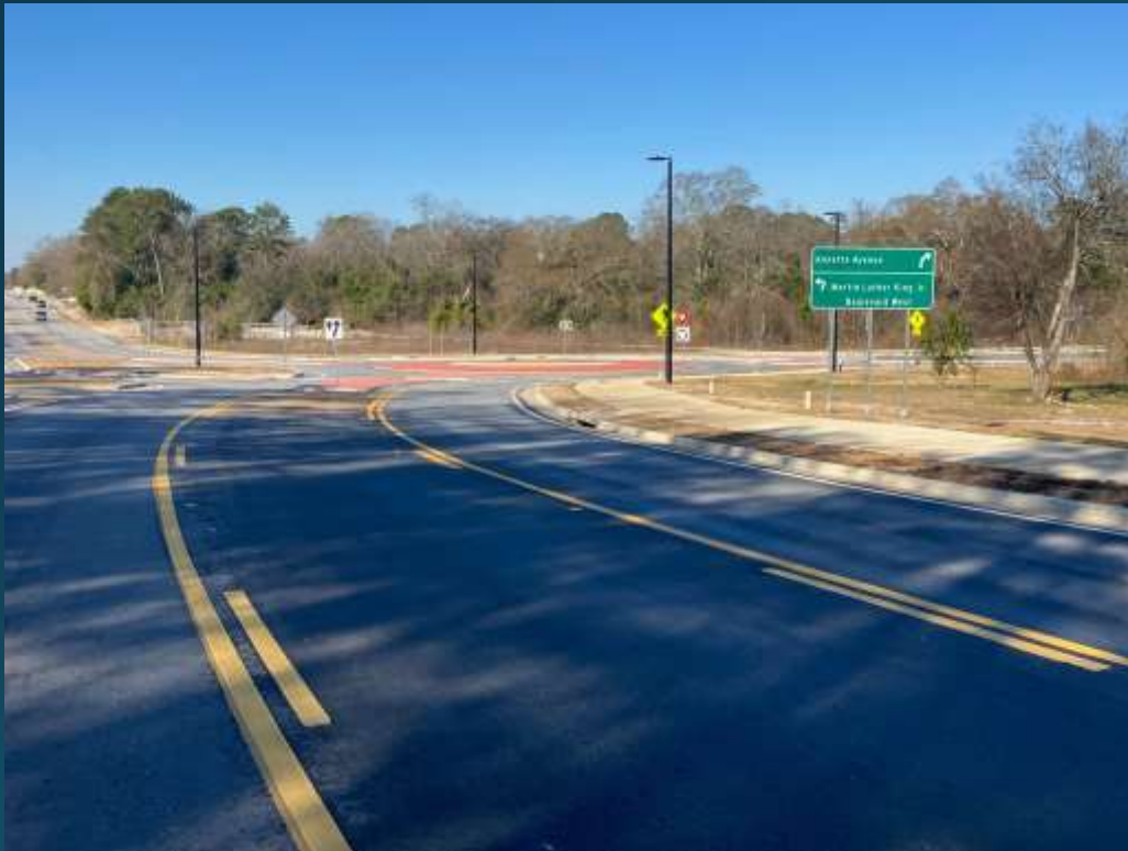
Phase I Roundabout
