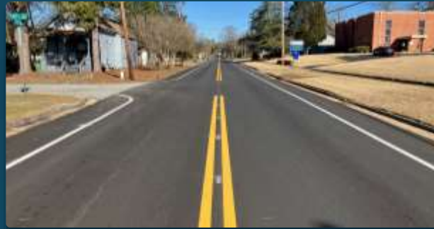
12 th Avenue Resurfacing/Striping
