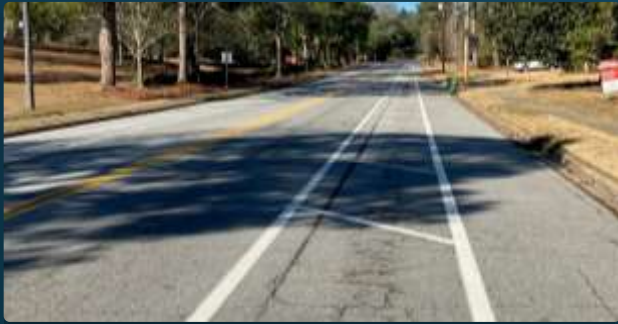
Edgewood Road Striping
