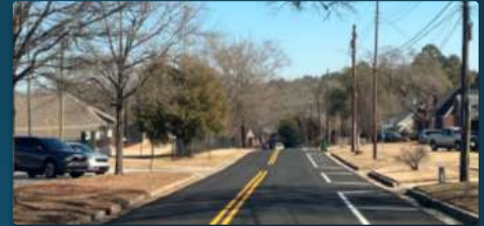
32 nd Street Resurfacing/Striping
