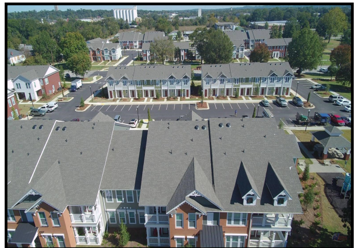
Aerial view of Arbor Point Apartments
