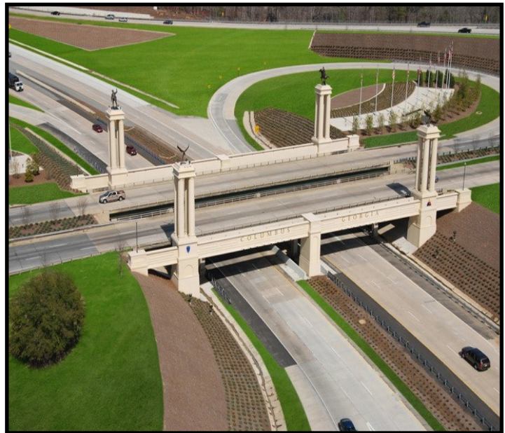
Fort Benning Gateway Bridge
