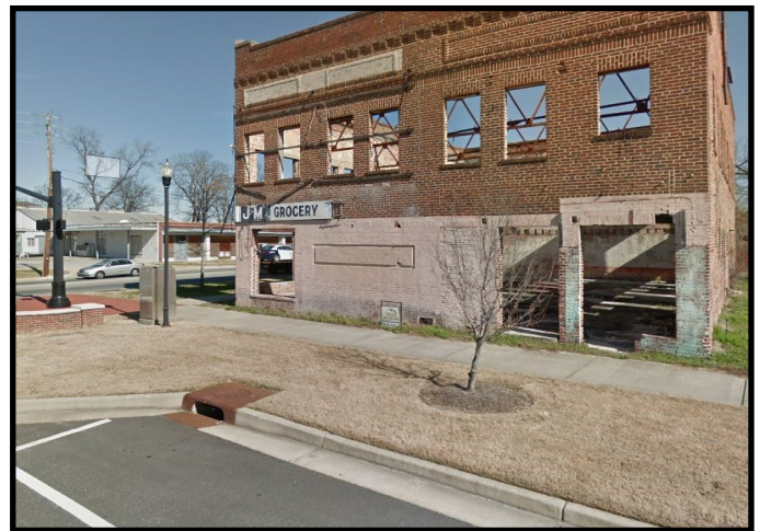
Dilapidated building along 6th Avenue
