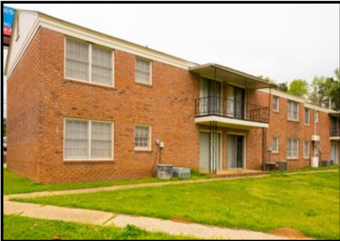
Apartments along Victory Drive
