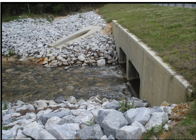
Lindsey Creek passing through a culvert
