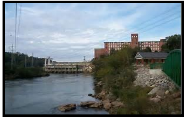
NORTH HIGHLAND DAM
