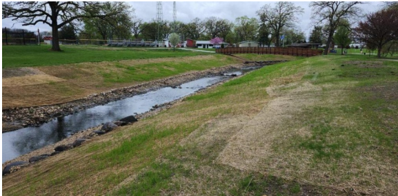
2025 Fireman's Park Culvert Removal
