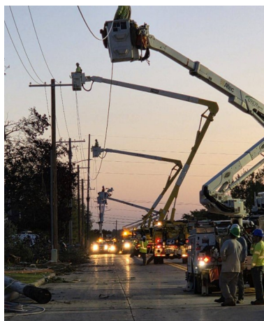
Mutual aid crews strung a three-phase feeder after multiple poles had to be replaced when tornadoes hit Juneau in May.
