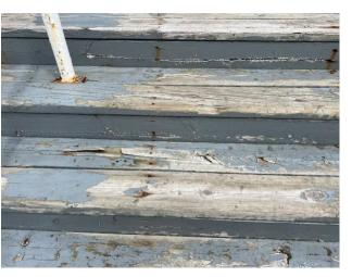
Wood treads contain exposed nails and splintered
