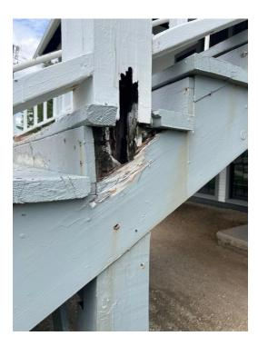
Areas of wood decay identified, though the structure is still sound
