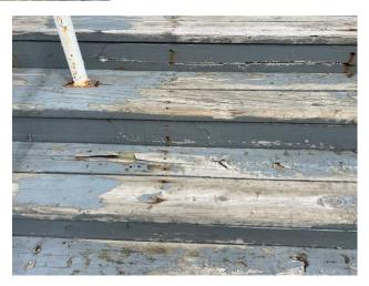
Wood treads contain exposed nails and splintered
