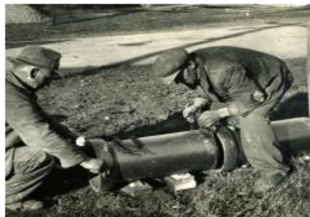
SETTING A NEW LATERAL.—1950's.
