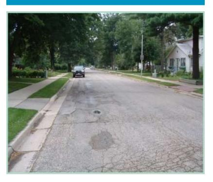
Severe rutting over 2" caused by poor mix design.
