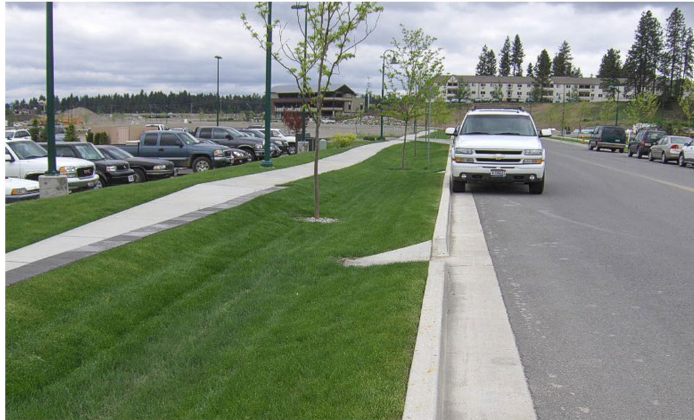
Photo courtesy of New Jersey Developers Green Infrastructure Guide (Keltic Engineering, Inc.)
