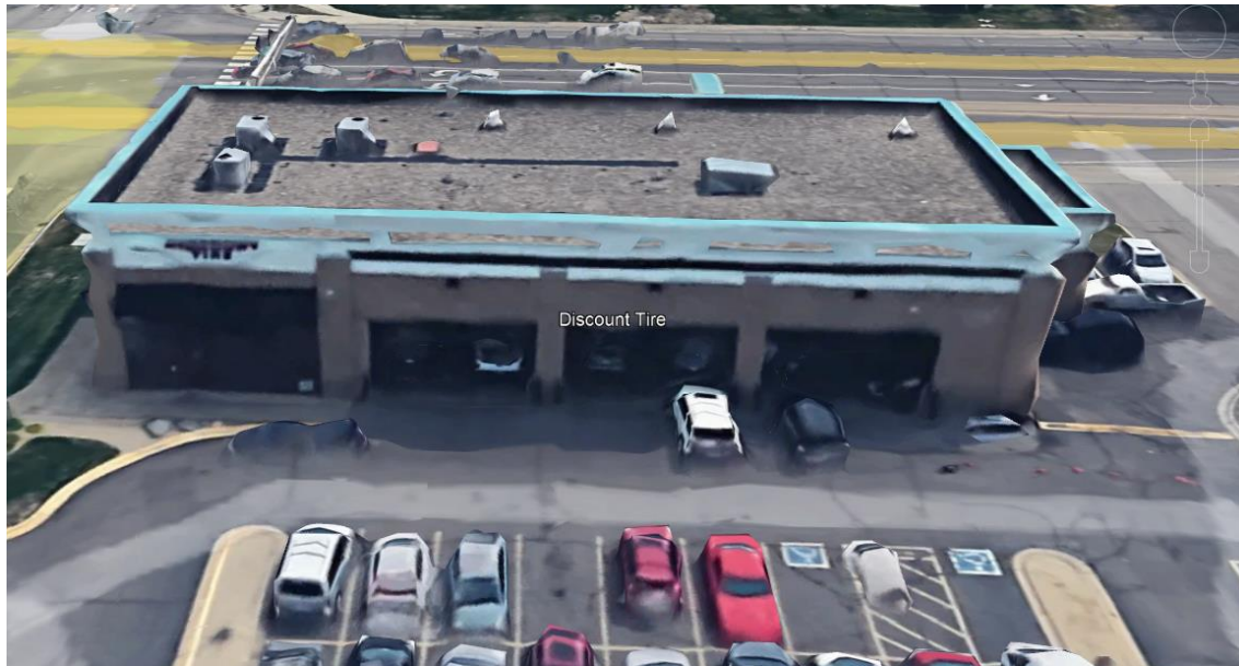
Discount Tires – Rooftop View
