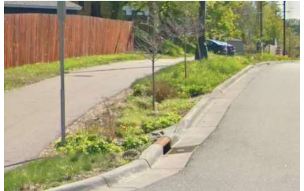
Stormwater infiltration basins on 37 th Ave
