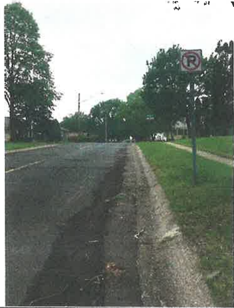
41 st looking west toward Monroe with showing incline
