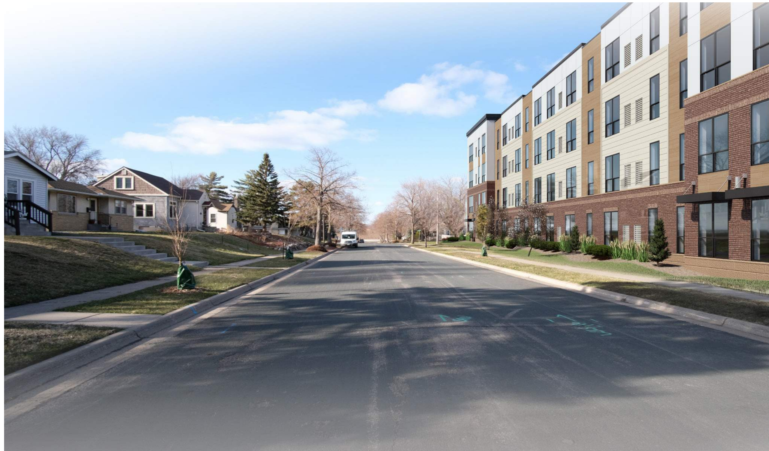
VIEW NORTH ON JACKSON ST NE
