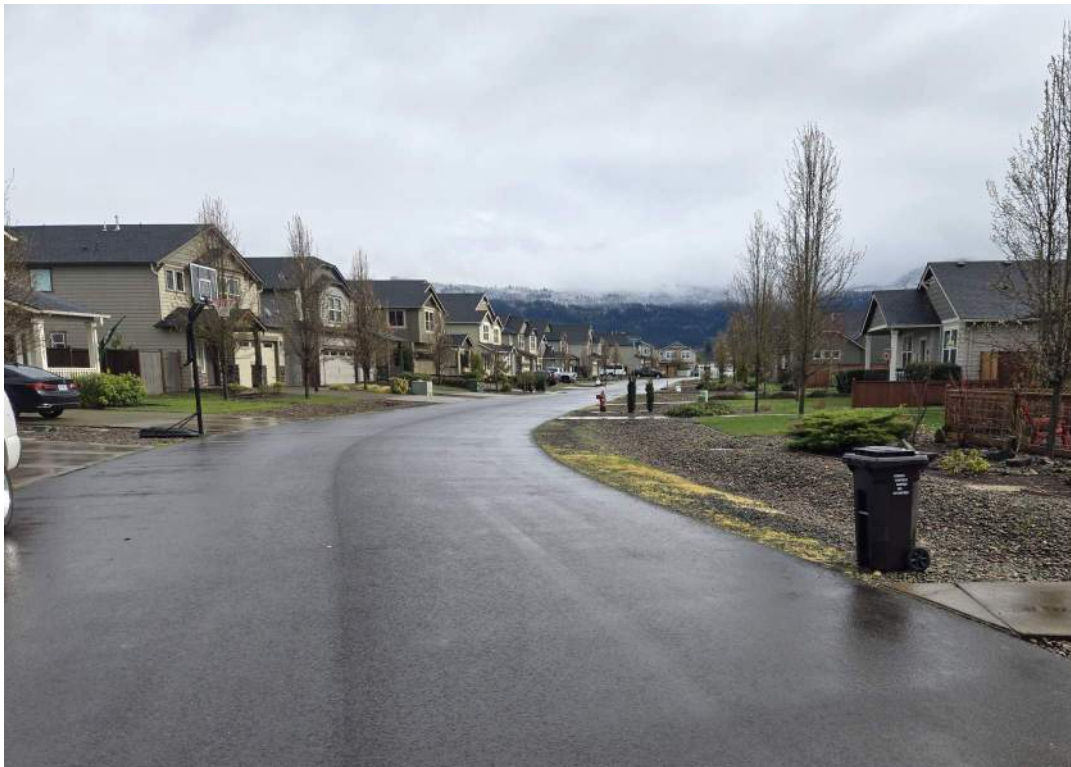
Figure 53: Coburg Crossing roadside stormwater facilities in 2024.
