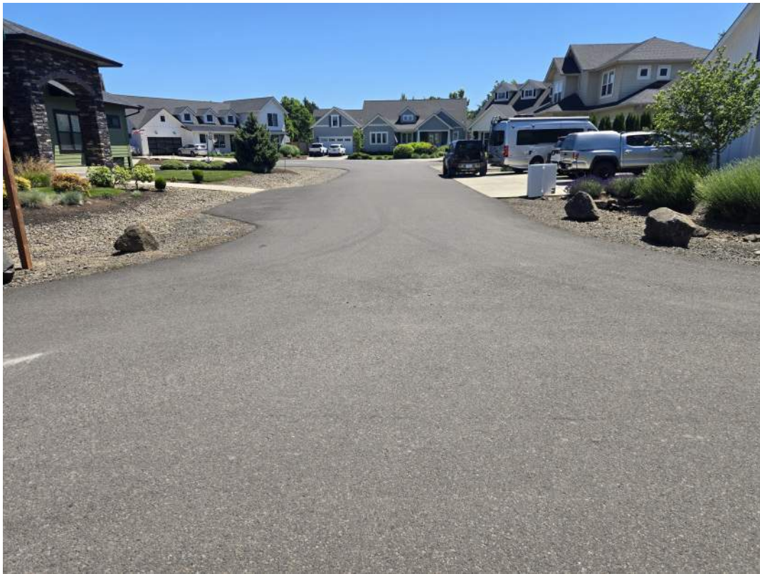
Figure 49: Hatfield Estates roadside stormwater facilities in 2024.
