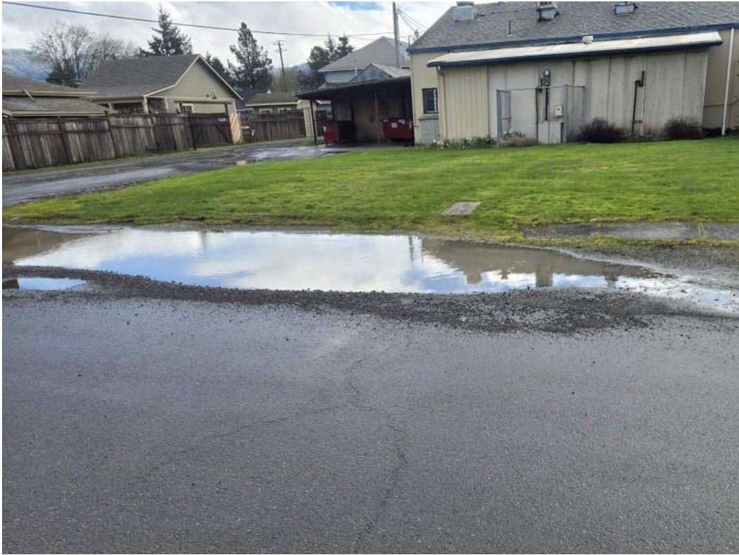
Figure 82: E. Locust St. looking at the Dari Mart in 2024.
