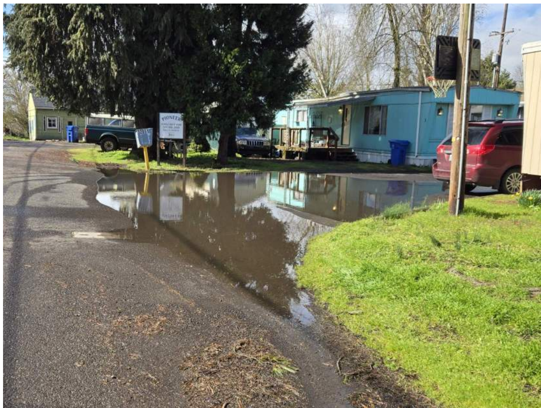
Figure 68: Ponding water at Pioneer Mobile Home Park in 2024.
