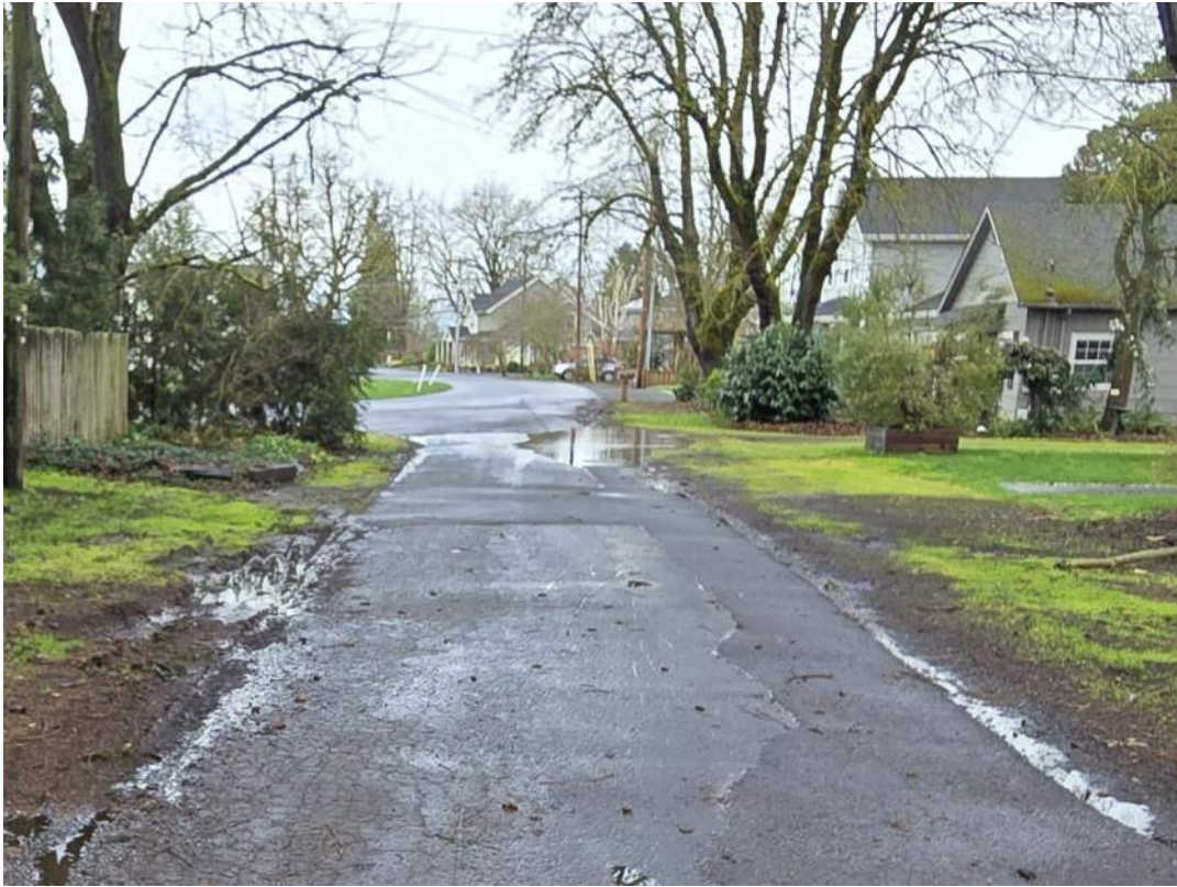
Figure 80: E. Locust St. looking west at N. Diamond St. in 2024.
