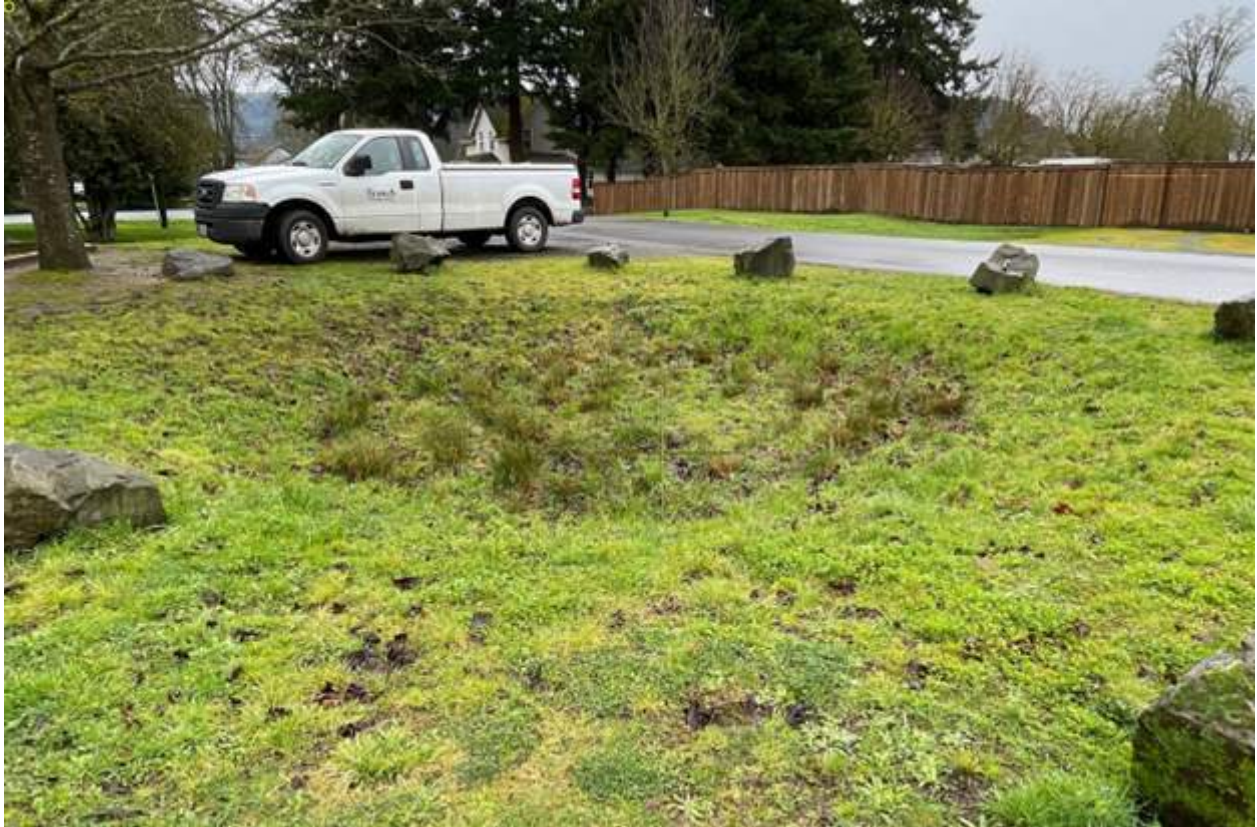
Figure 35: Rain garden at the northeast corner of McKenzie and Harrison, constructed during the intersection reconstruction project. Photo taken in 2021.
