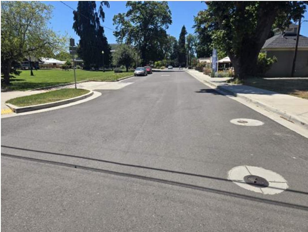
Figure 38: McKenzie St. in 2024, after the reconstruction project.
