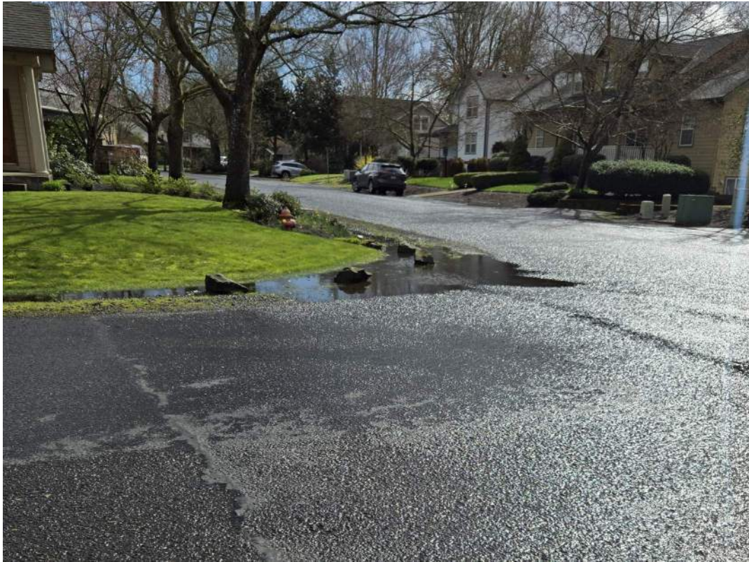
Figure 88: SE Corner of Austin Rd. and Abby Rd. infiltration deficiency in 2024.
