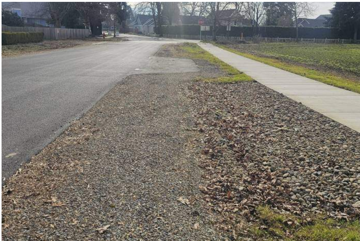
Figure 30: N. Willamette St. completed storm facility at construction completion in 2024.
