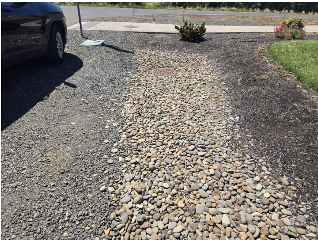
Figure 50: One of the two overflows at the west end of Hatfield St. in 2024.
