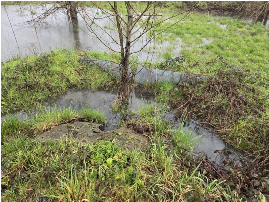
Figure 93: Coburg Industrial Way and Roberts Rd. retention basin inlet in 2024.
