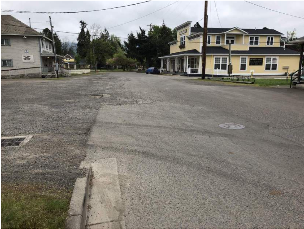
Figure 43: South side of Mill St. taken in 2018 from the west, prior to 2018 reconstruction project.
