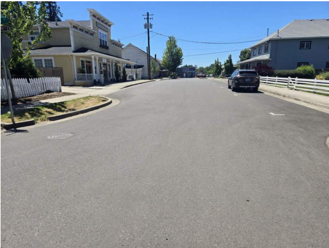
Figure 44: Mill Street in 2024, after the reconstruction project.
