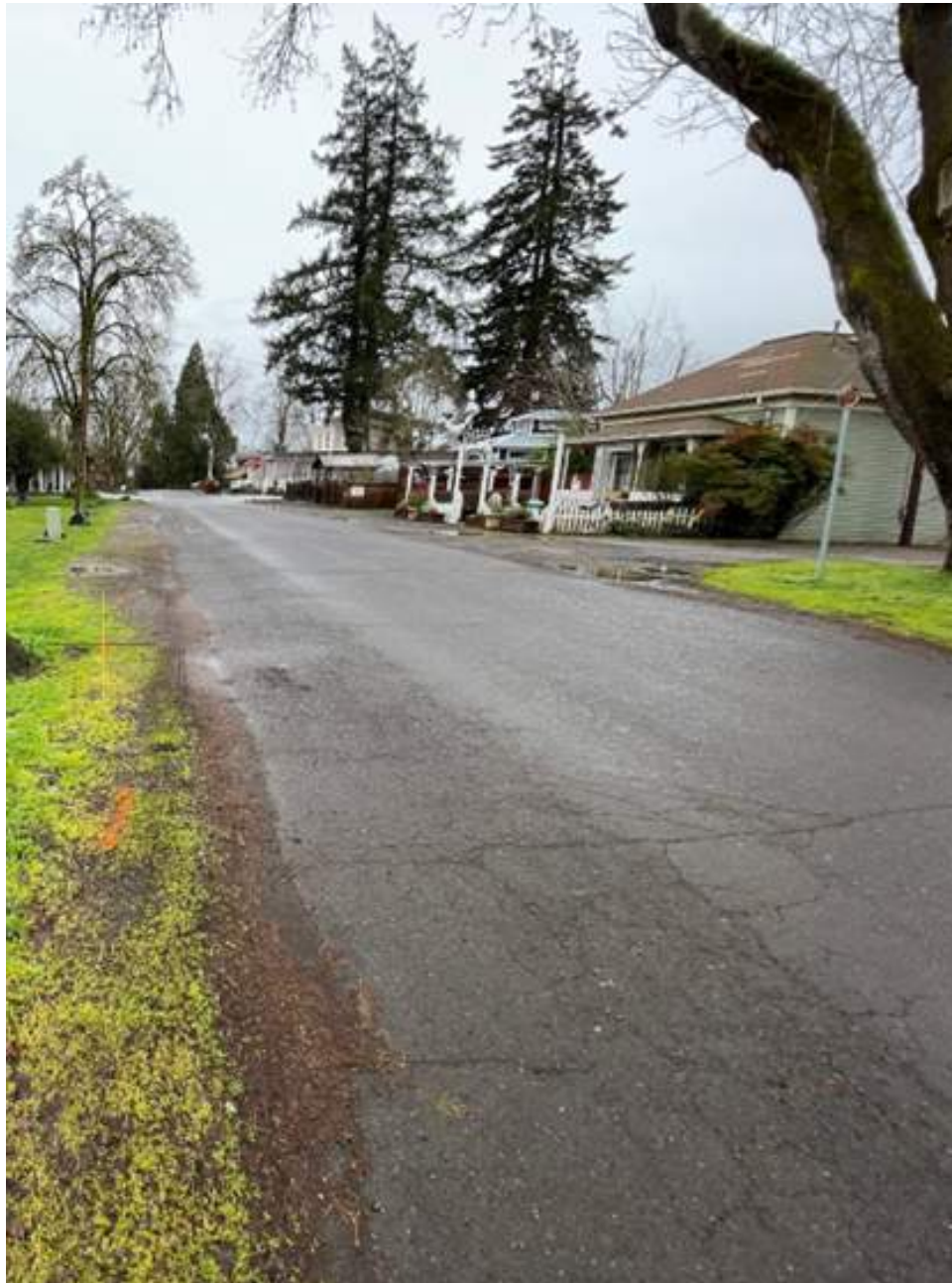
Figure 36: McKenzie St. in 2021, prior to the 2022 reconstruction project.
