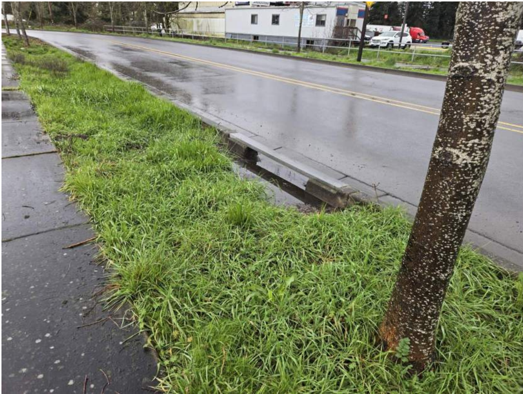
Figure 90: Coburg Industrial Way curb inlet in 2024.
