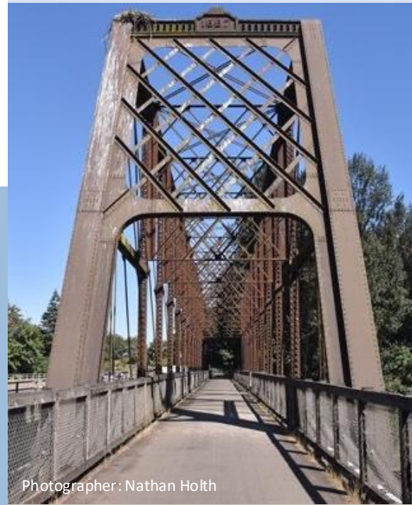
Armitage Bridge Coburg, OR
