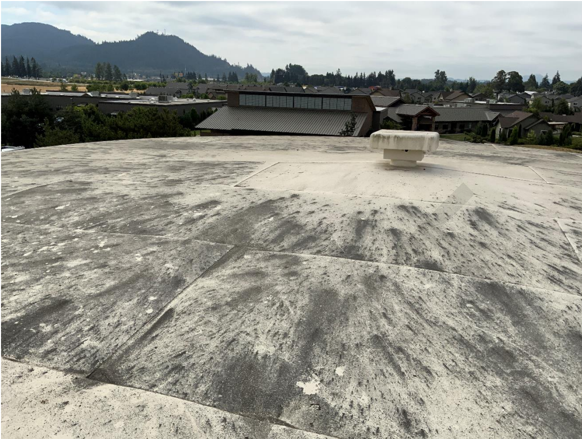
Photo 21 – Tank Exterior Roof
