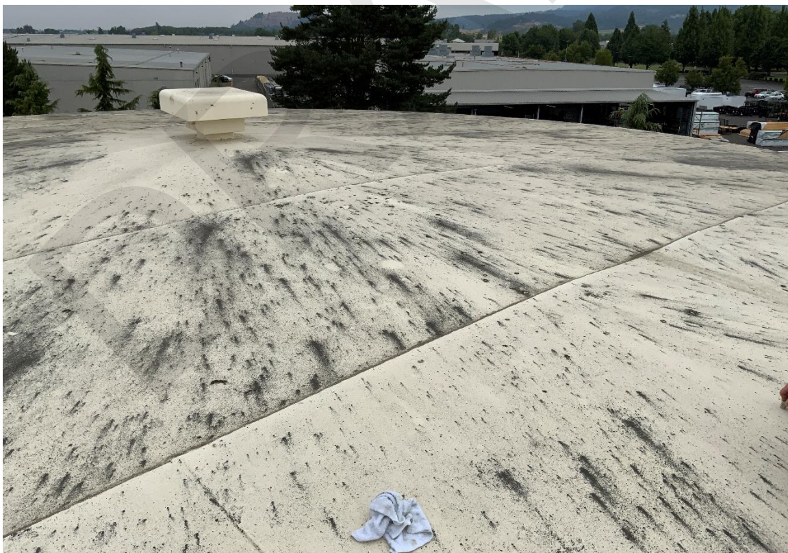
Photo 8 – Tank Exterior Roof
