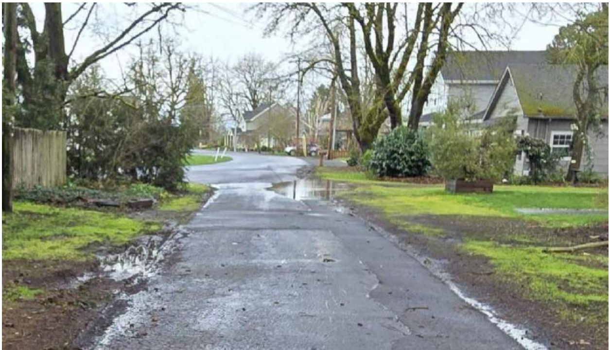
Figure 7: Ponded water on E. Locust St. due to deficient roadside infiltration, looking west to N. Diamond St.
