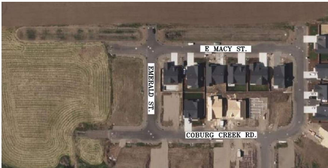
Figure 2: Detention swales in NW of Coburg, with overflow to Mill Slough
