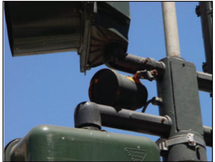
Audio signal at signalized intersection tells pedestrians when it is safe to cross.
