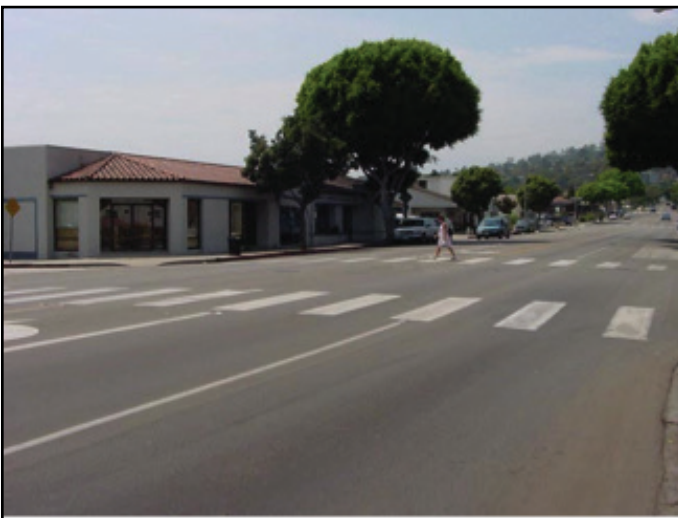
Continental-style marked crosswalk at midblock crossing is visible from farther away
