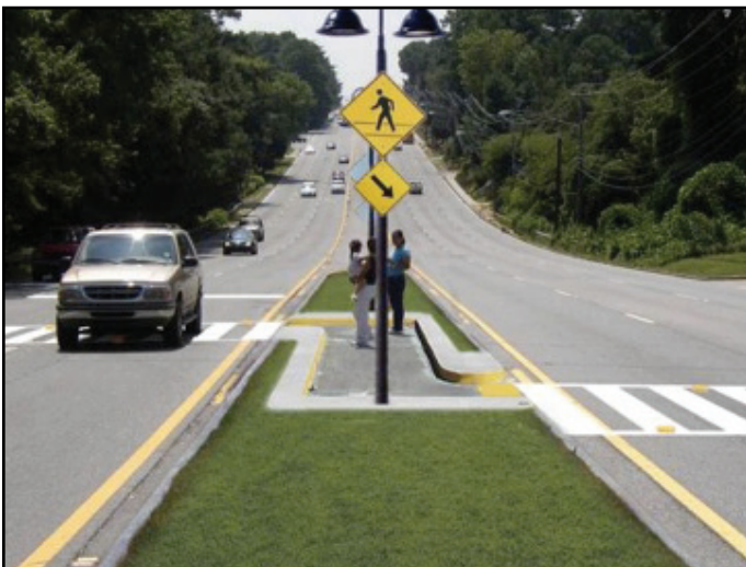
A gap and channelization in this raised median places pedestrians in correct orientation to cross
