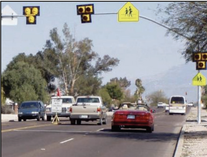
Pedestrian hybrid beacon on four lane street with high speeds and volumes
