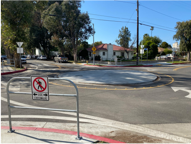
Alta led the design for a neighborhood traffic circle for LADOT's Sherman Way Streetscape improvements.
