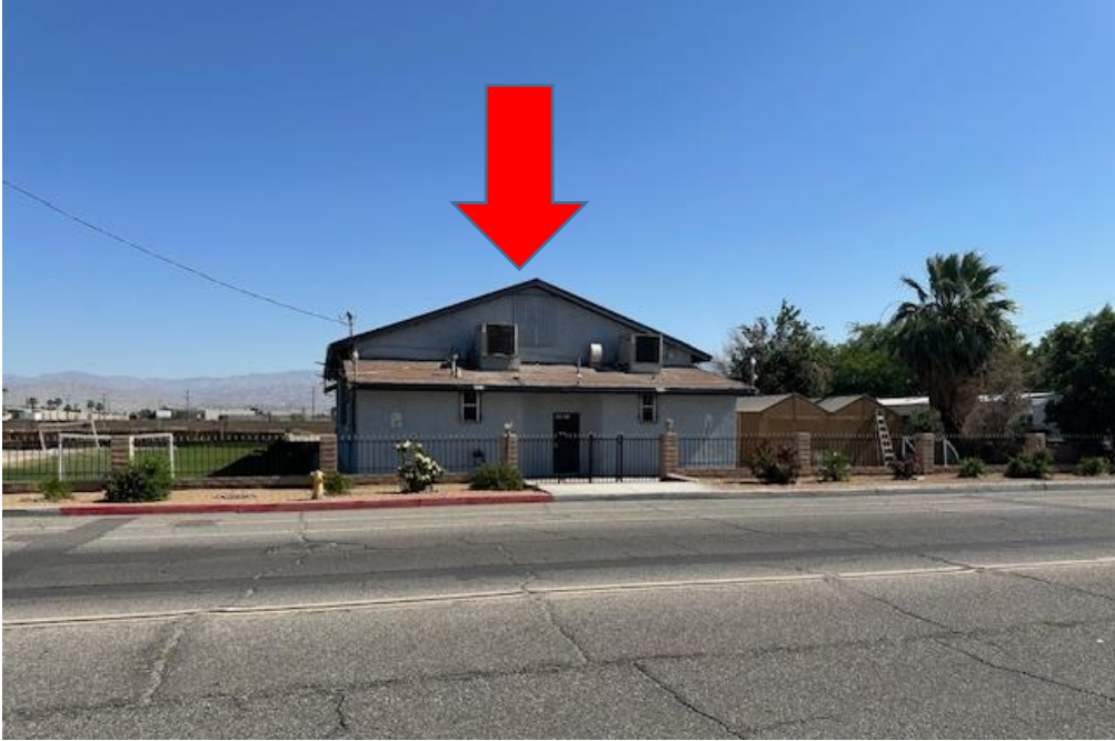
Existing Mosque Front View
