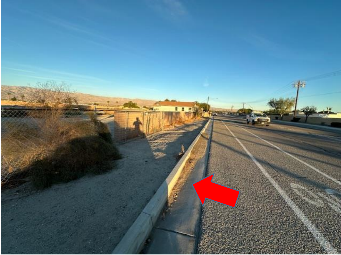
Existing Avenue 49 Landscaping
