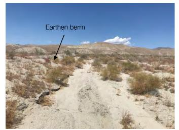
Photo 35. Upstream view of Feature 8 flowing south parallel to the earthen berm, which stops flows from continuing further west and instead directs them south towards a highway undercrossing. Photo taken facing northeast. May 7, 2019.
