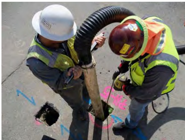
C Below technicians performing potholing
