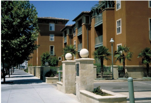
Three-story apartment complex with a landscaped setback.
