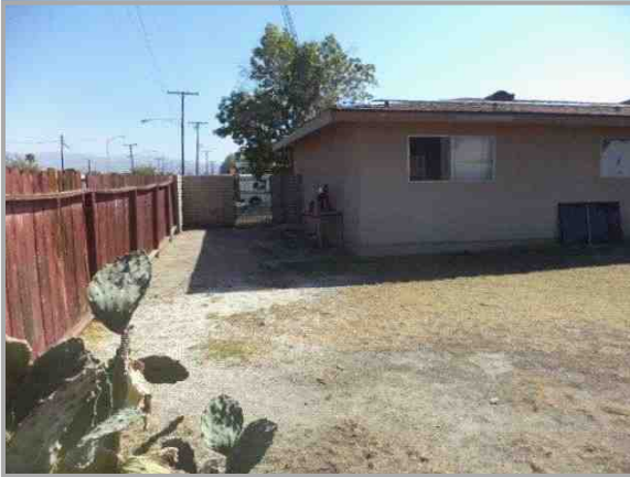
Rear and north side
