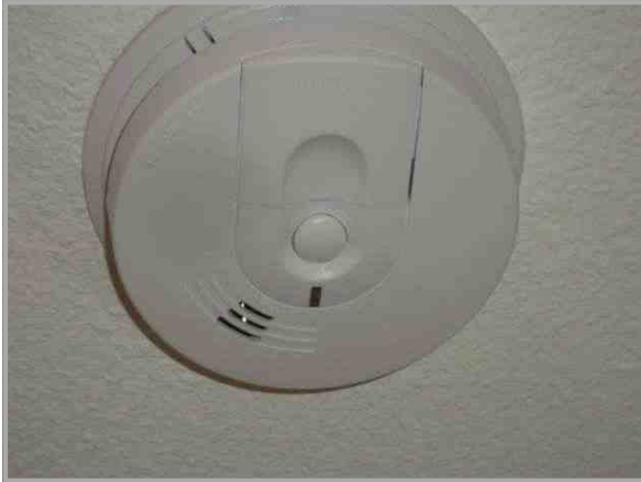
Combined CO2 detector and smoke alarm
