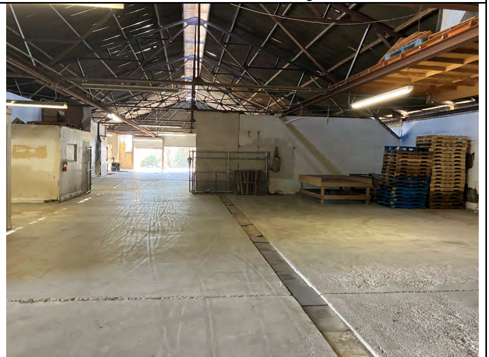
Photo No. 16 – Southeast view of building's central interior area.
