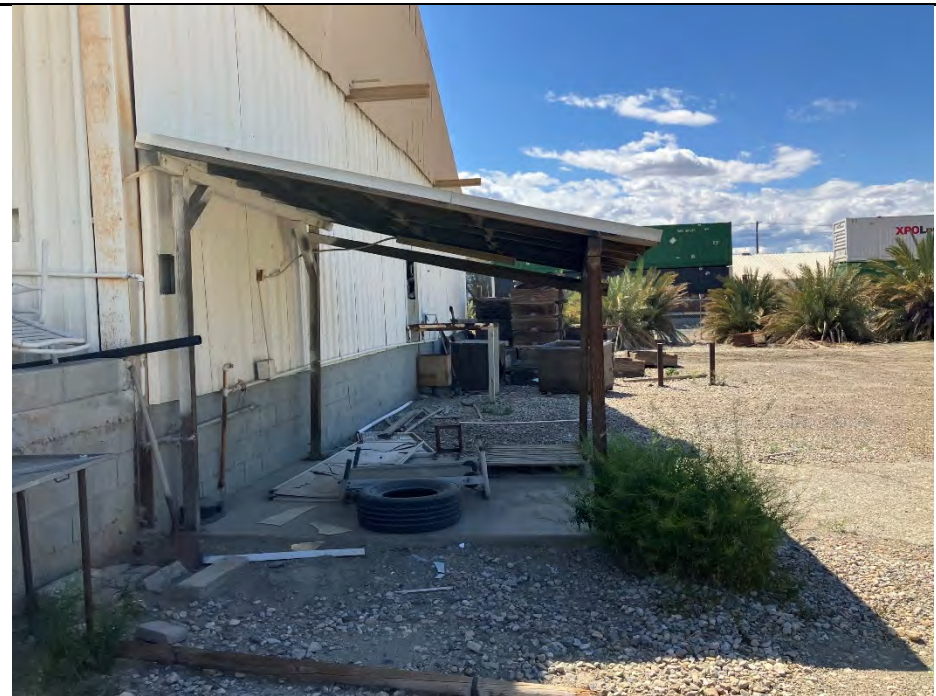
Photo No. 6 – Southwest view of building's northern side.
