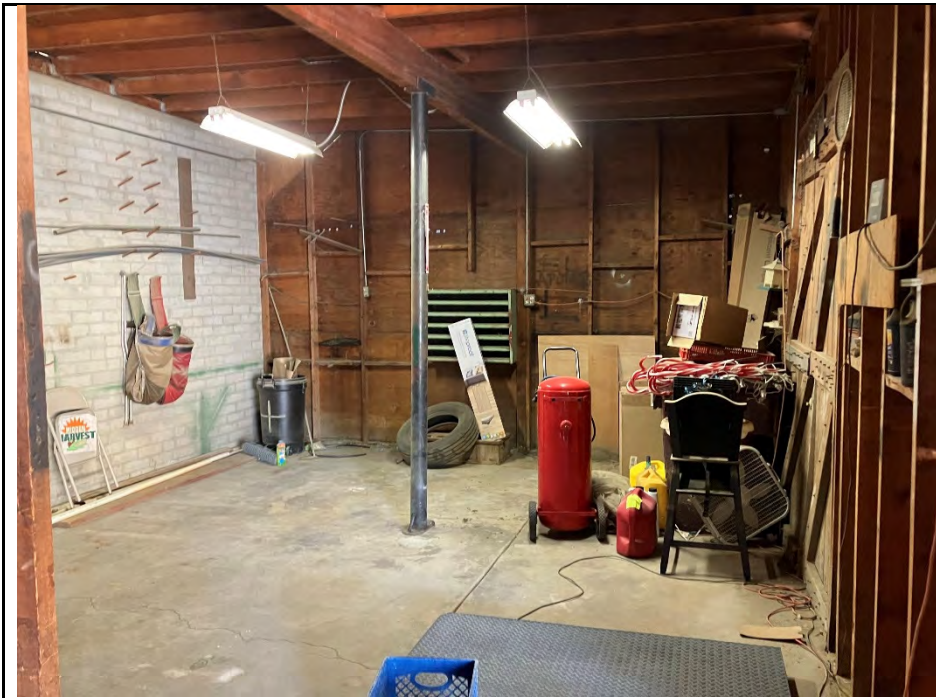
Photo No. 13 – Northwest view of room in building's southern portion.
