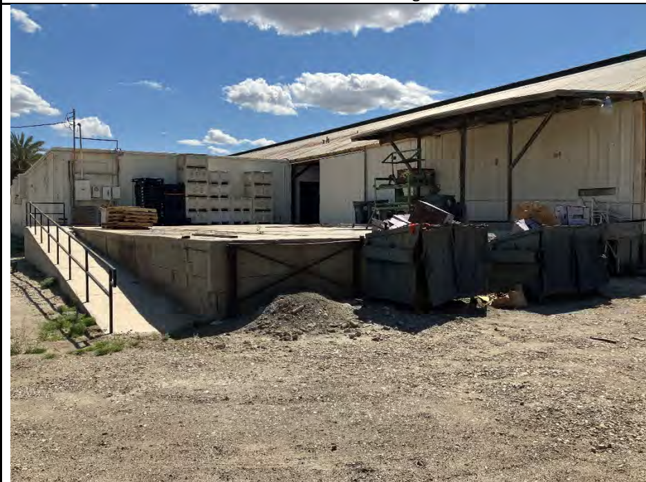
Photo No. 7 – South view of loading dock.
