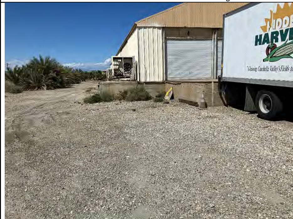
Photo No. 3 – Northwest view of loading dock.
