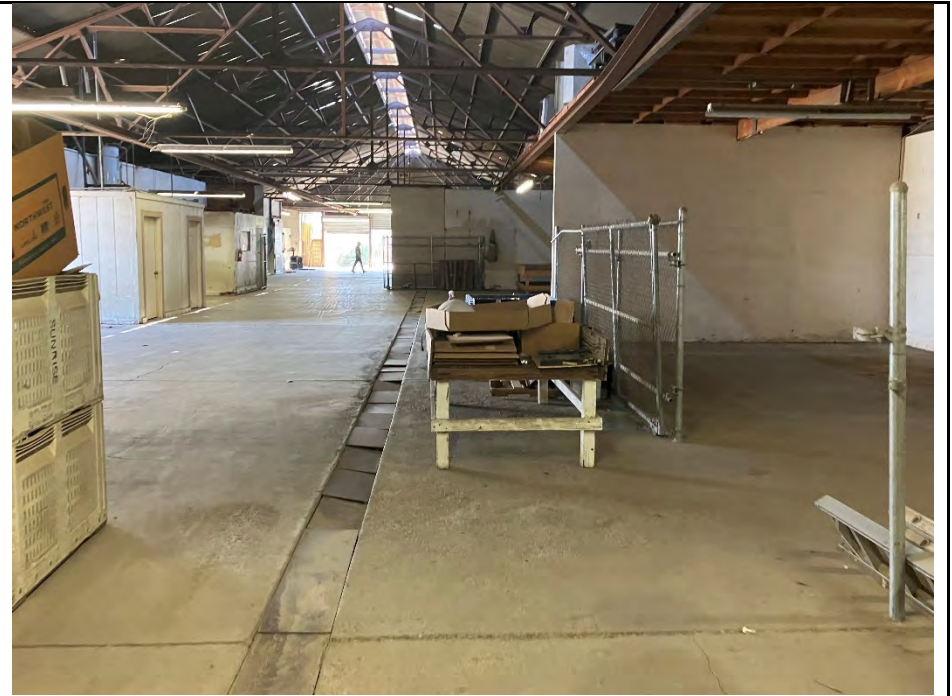
Photo No. 18 – Southeast view of building's northern interior area.
