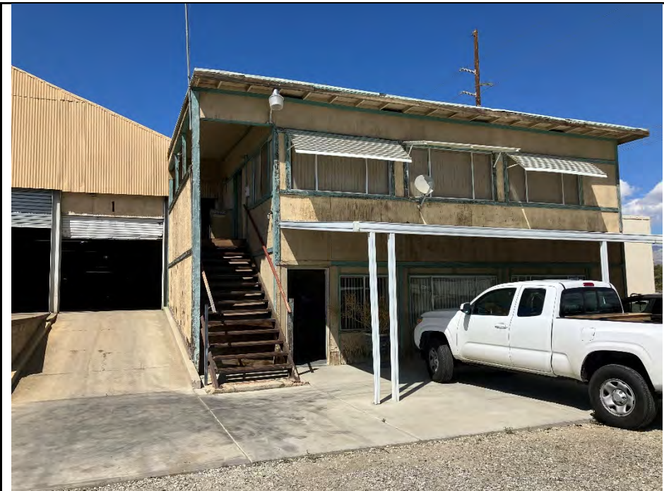
Photo No. 2 – North view of office and kitchen area.
