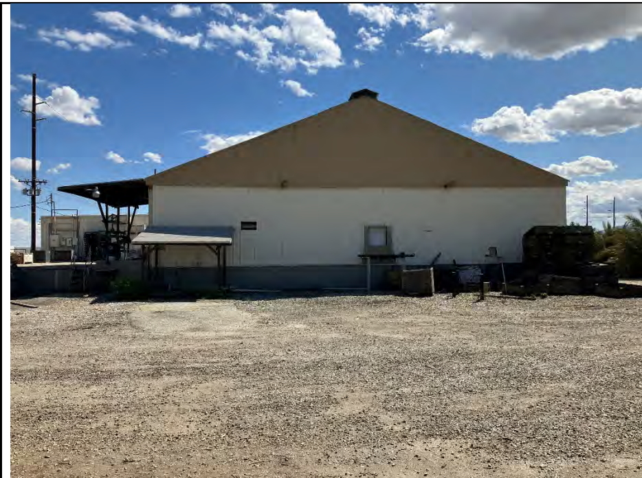
Photo No. 5 – Southeast view of building's northern side.
