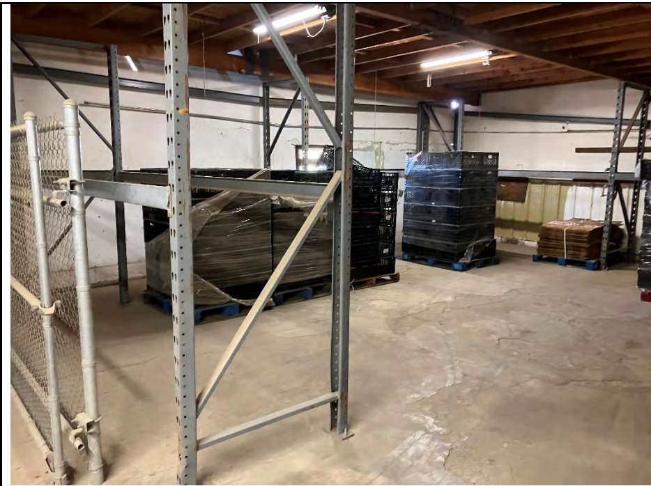
Photo No. 21 – Northeast view of room in building's northeastern portion.
