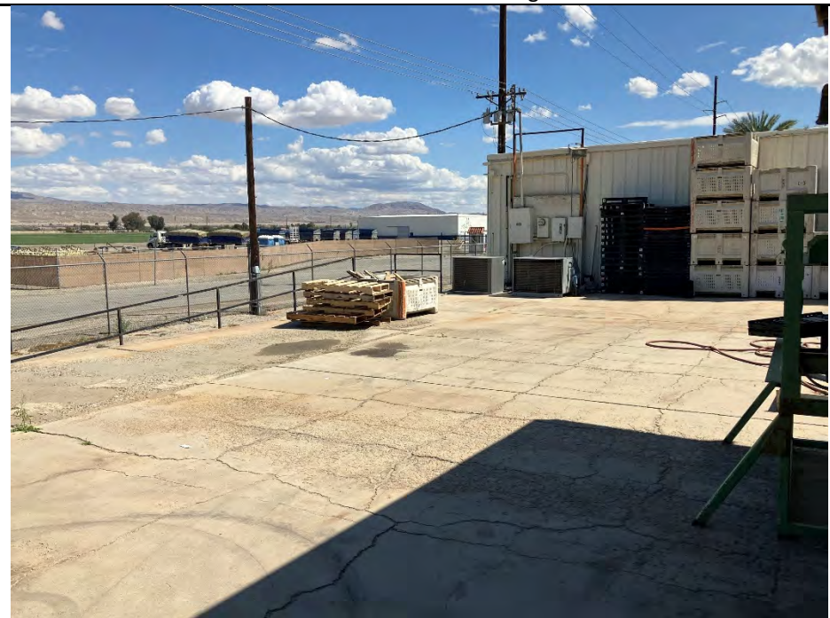
Photo No. 8 – Southeast view of loading dock.
