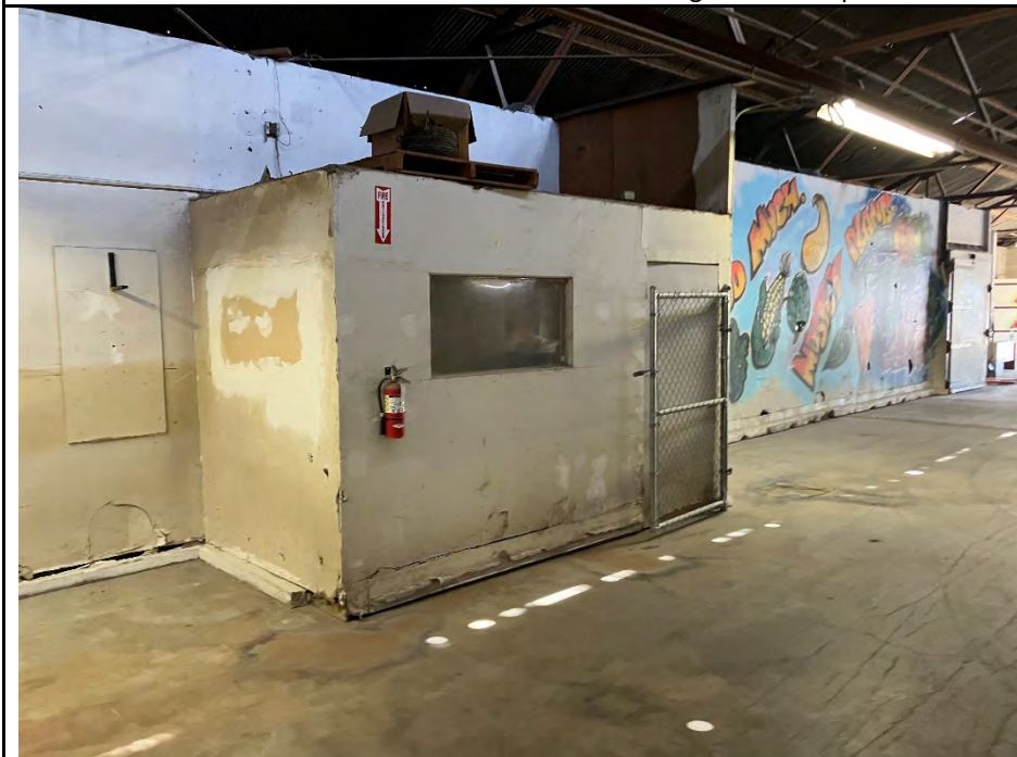
Photo No. 15 – Southeast view of building's central interior area.
