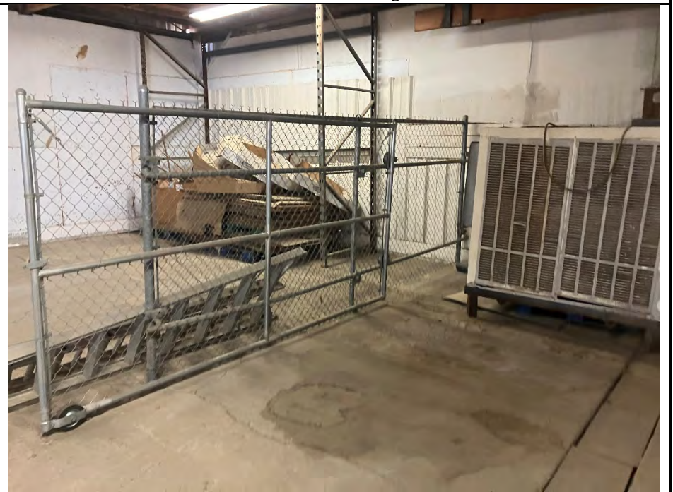
Photo No. 20 – Northwest view of building's northern interior area.
