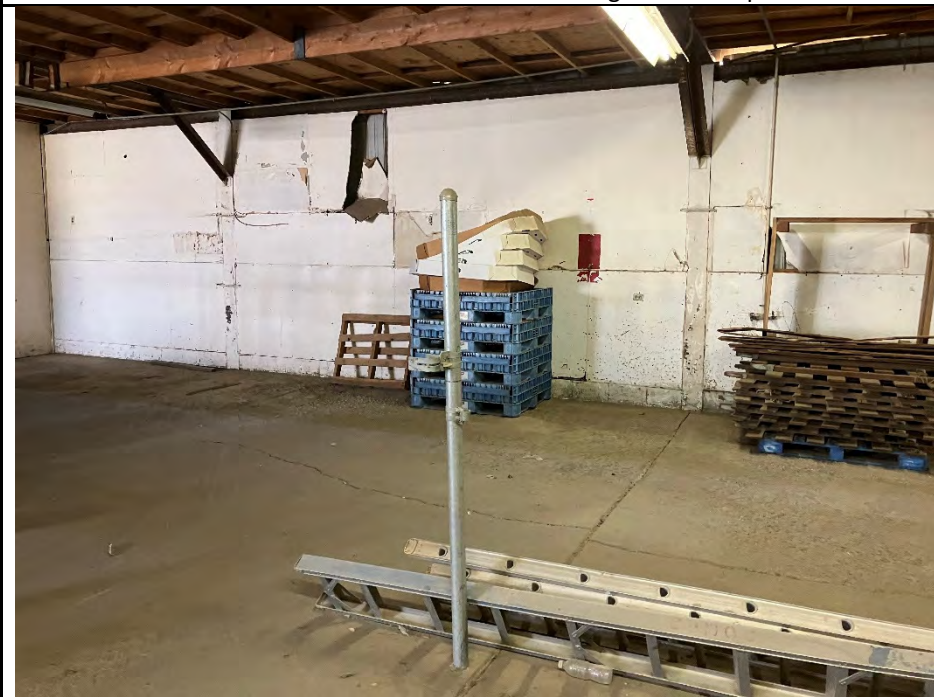
Photo No. 19 – Southwest view of building's northern interior area.
