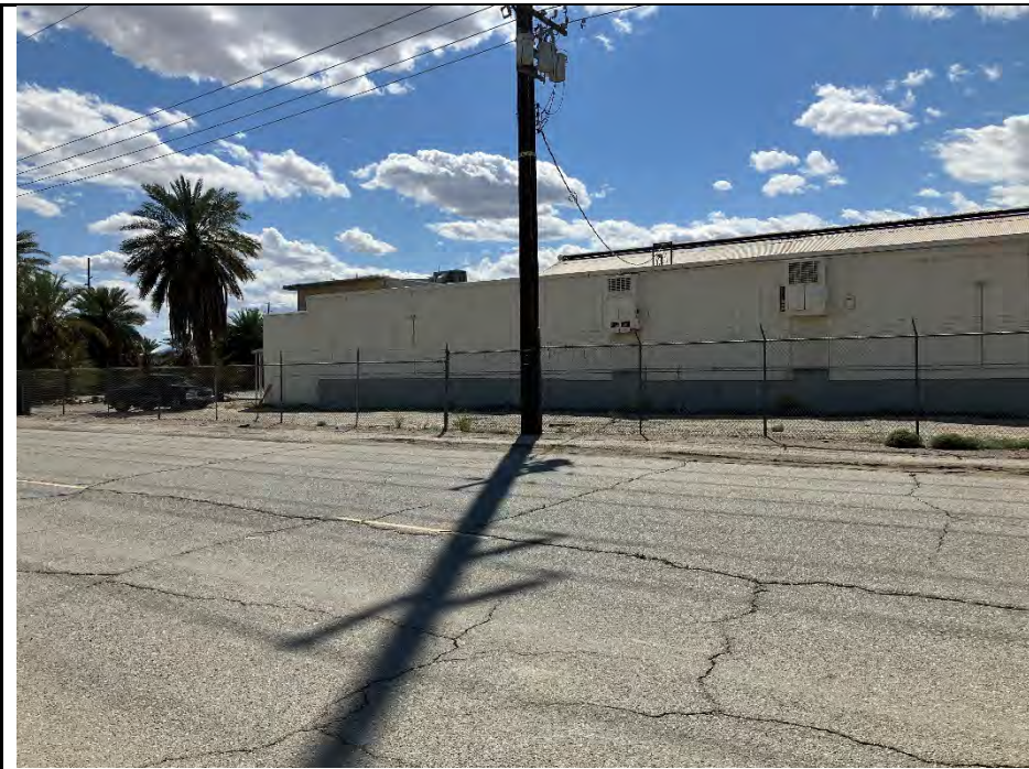
Photo No. 9 – South view of building's eastern side.
