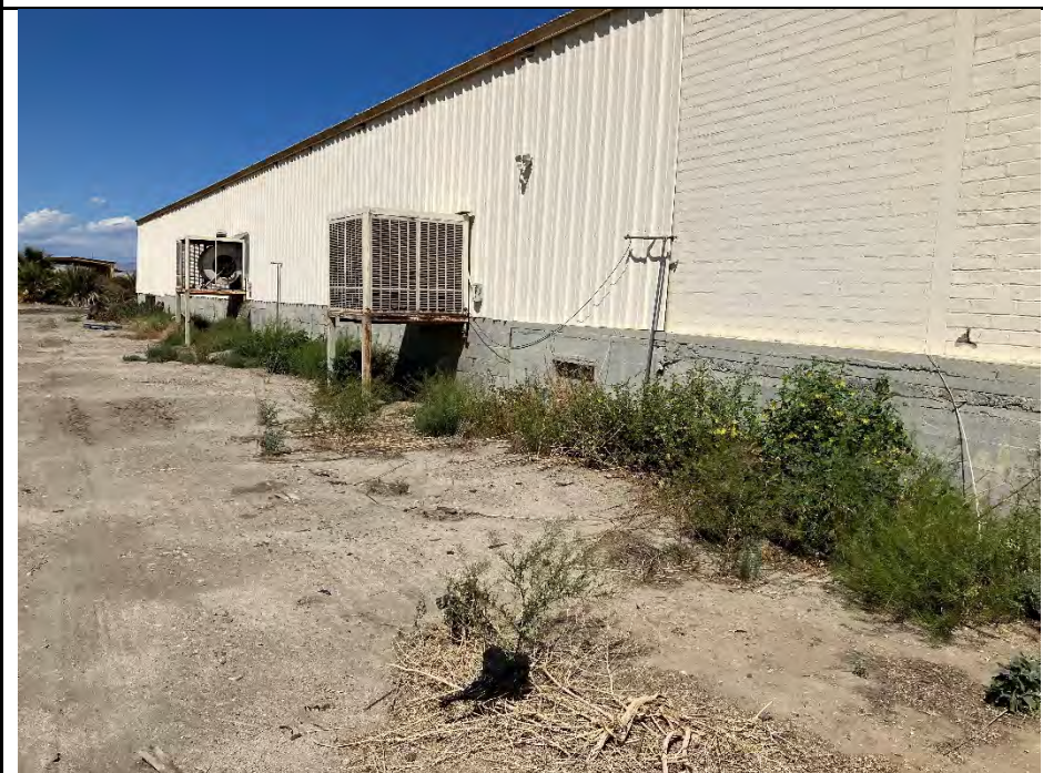
Photo No. 4 – North view of building's western side.
