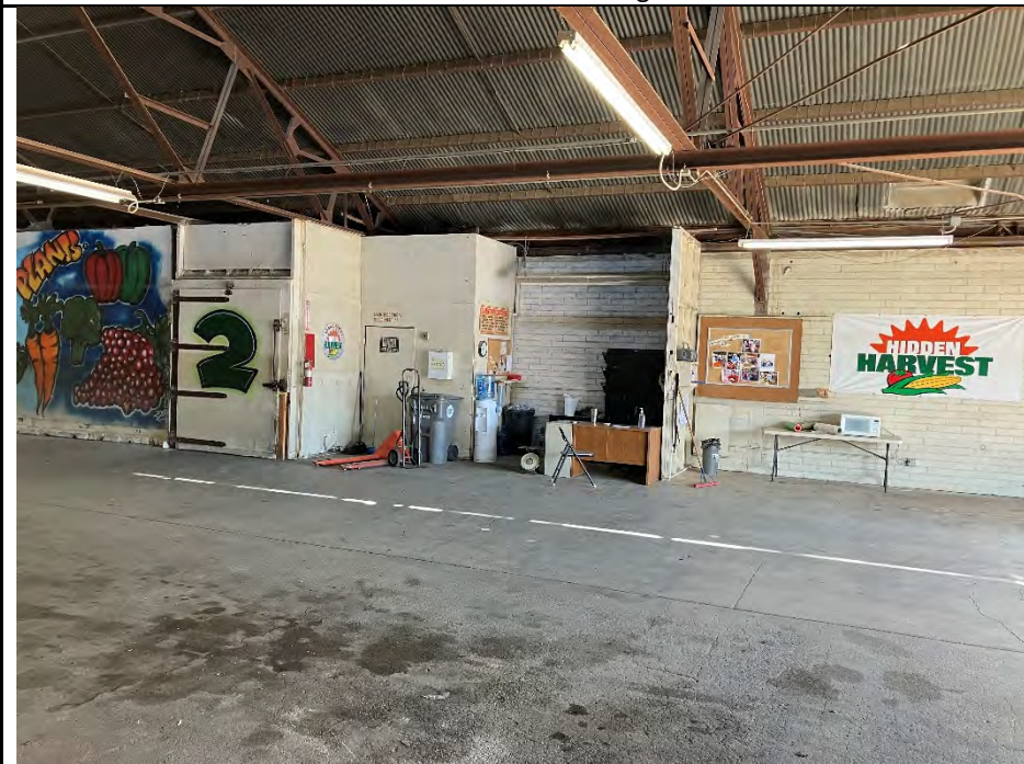
Photo No. 11 – North view of building's southern interior area.
