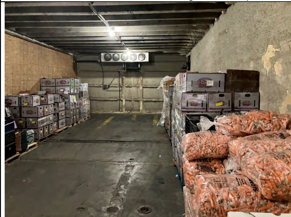
Photo No. 23 – Northeast view of Cooler No. 2 (southern half only).
