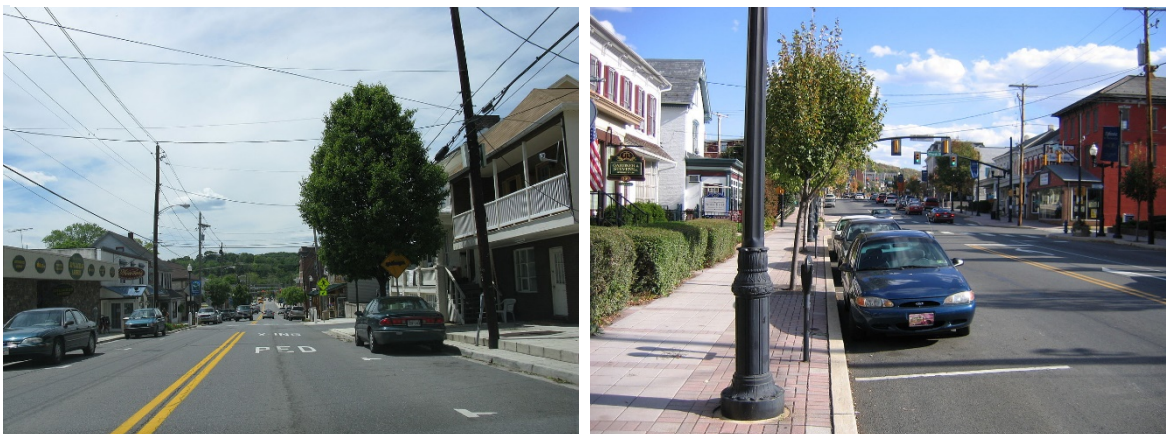
On Street Parking and Lane Making Giving Perception of Reduced Lane Width. SOURCE: Andrew Bossi
