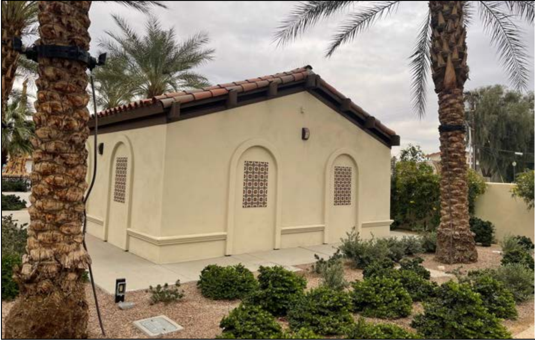
Rear of the Veteran's Park restroom buildings.
