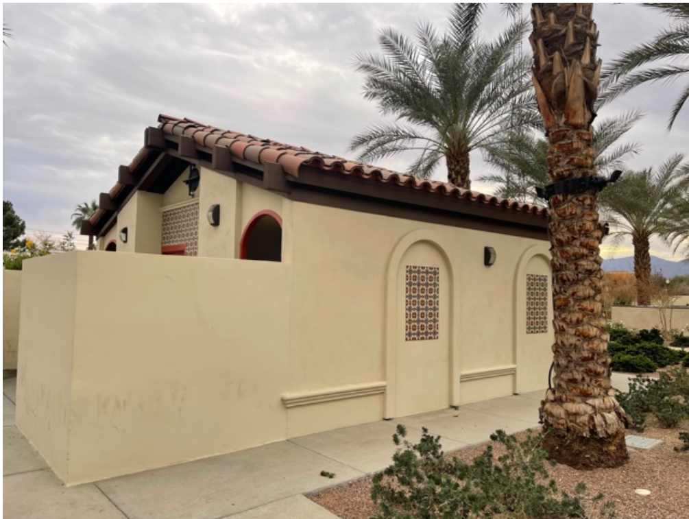
Restroom at Veteran's Park with smooth stucco, tile accents, exposed rafter tails, grates and rounded doors.
