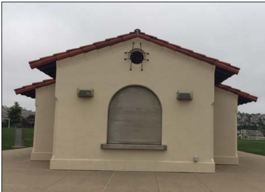
Example of an Ancillary Municipal Snack building with the slaking of the stucco at the edge of the tile roof.
