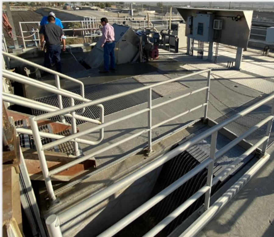
Figure 1. Existing Headworks Platform
