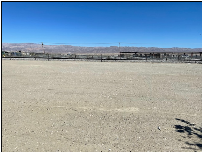
On-site improvements- Site groundcover with compacted decomposed granite for event area and parking.
