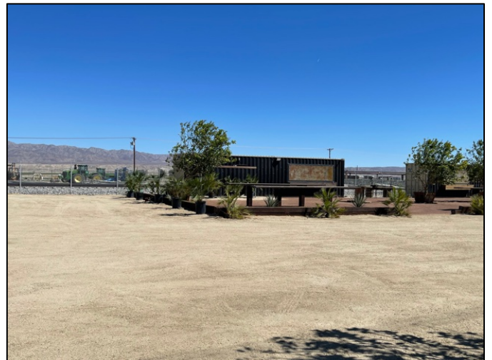
On-site improvements- Site groundcover with compacted decomposed granite for event area and parking.
