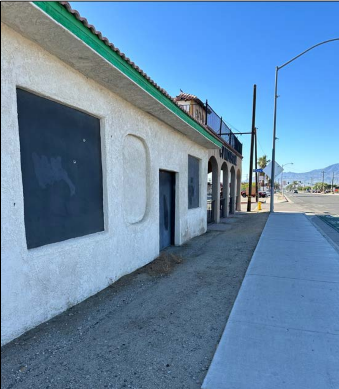
Front Building Façade facing Cesar Chavez Street
