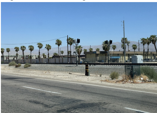
Existing swale and utilities in trail alignment
