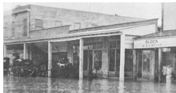
Classic Old West Architecture (Use of Colonnade)
