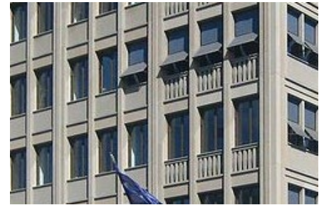
Balustrade and Use of Pilasters, Corner Treatment of Buildings. SOURCE: Jörg Zägel
