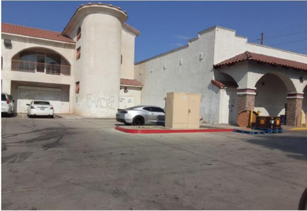
Photographs of Rear Parking Lot:
