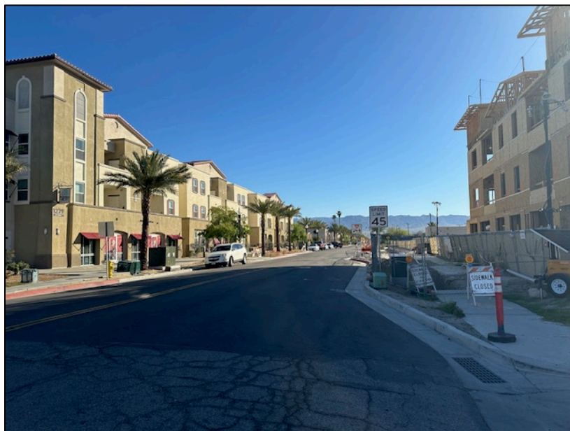
6 TH Street View looking East
