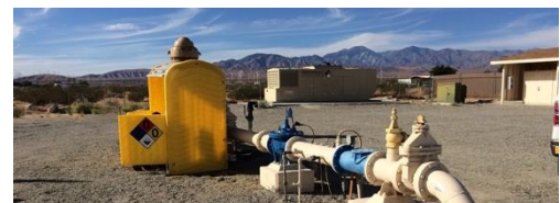
Figure 4. Corona directed full-scale demonstration of stannous chloride without filtration at CVWD ID-8 Sky Valley
