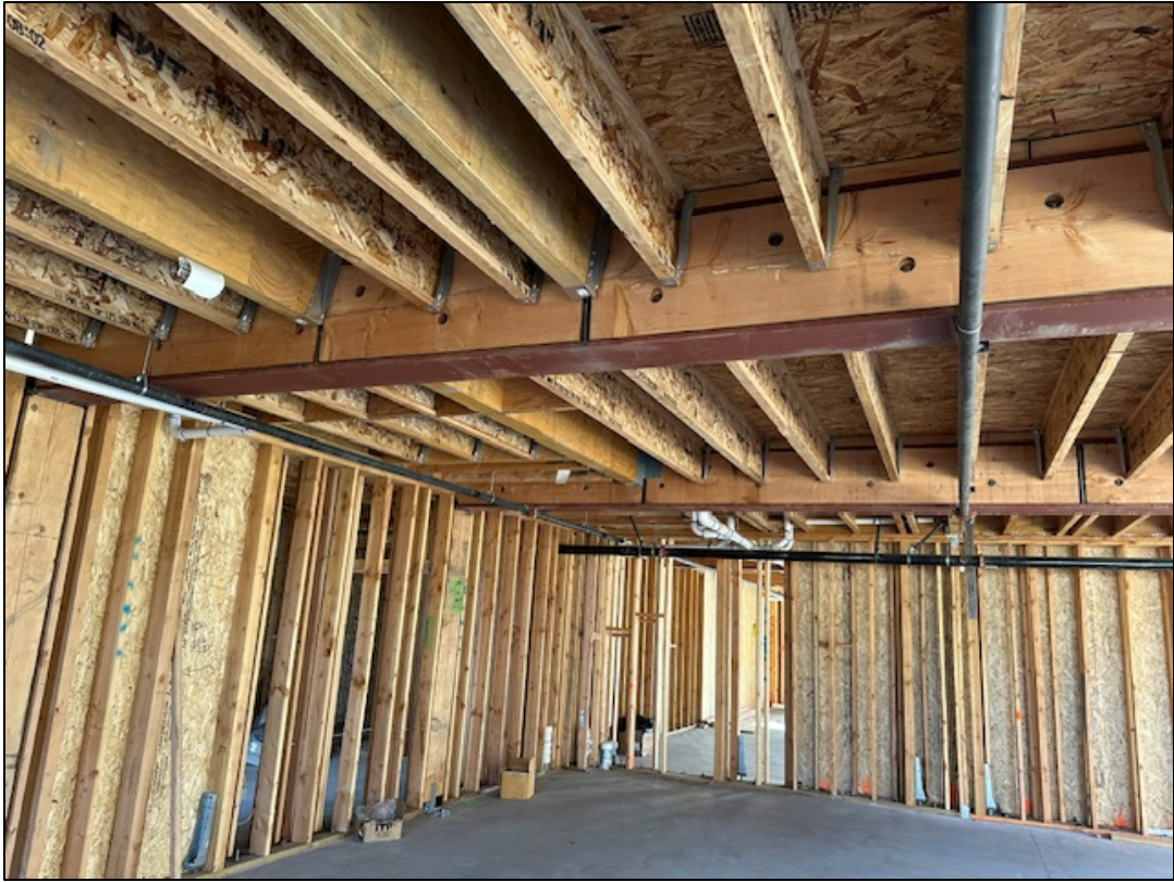
Unfinished Commercial Space in Covalda Apartments
