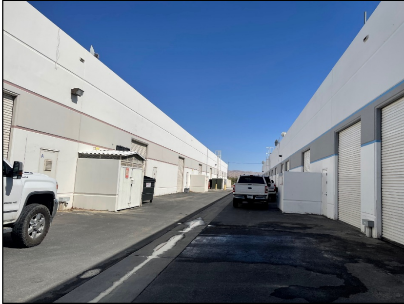
Rear Service Driveway
