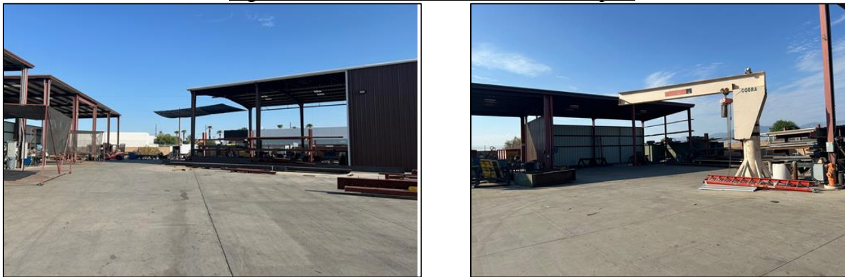
Figure 1 and 2: Photos of Site Metal Canopies
