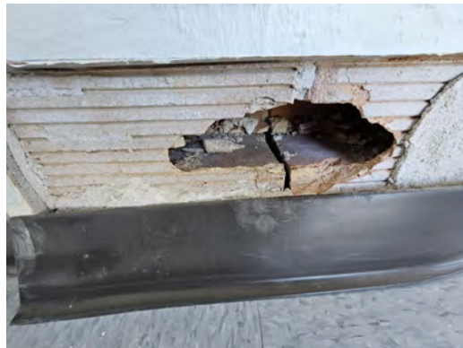
No reinforcement in clay/masonry walls
