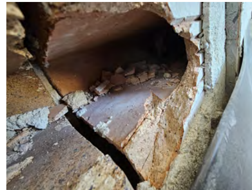
No reinforcement in clay/masonry walls
