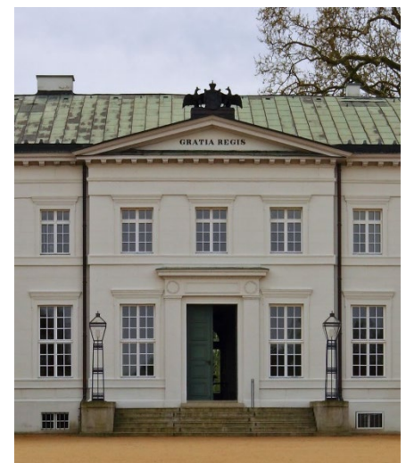
Vertical Proportioned Windows, Decorative Entryways, Pediment. SOURCE: A.Savin
