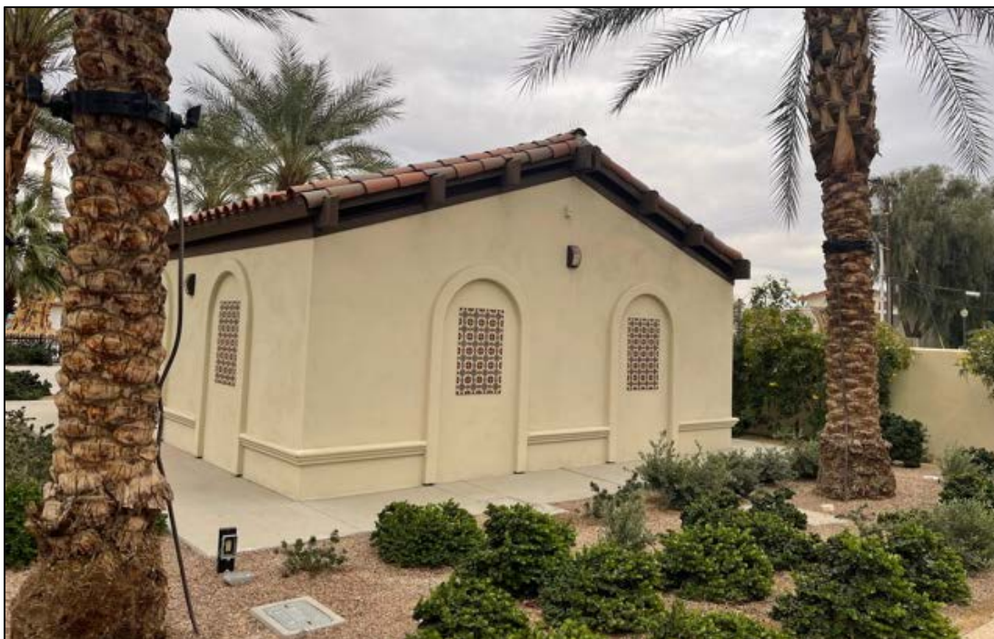
Rear of the Veteran's Park restroom buildings.
