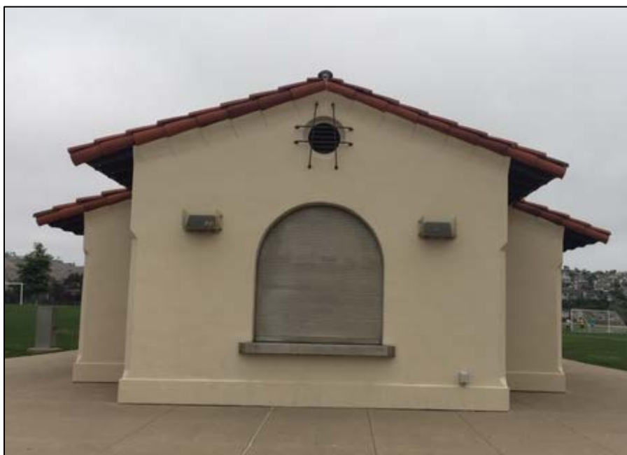
Example of an Ancillary Municipal Snack building with the slaking of the stucco at the edge of the tile roof.
