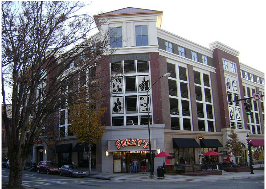
Programmable First Floor Space of Parking Garage. SOURCE: Michael Rivera
