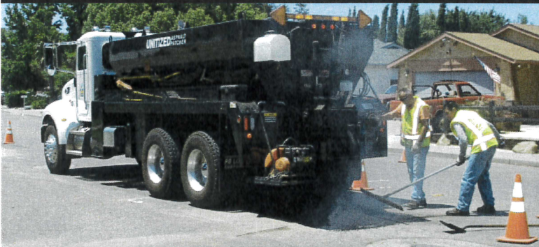
Compact asphalt material.
