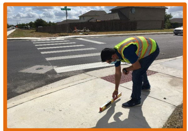
Performing a Crosswalk Inspection for ADA Compliance
