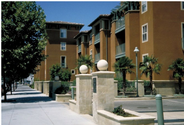
Three-story apartment complex with a landscaped setback.
