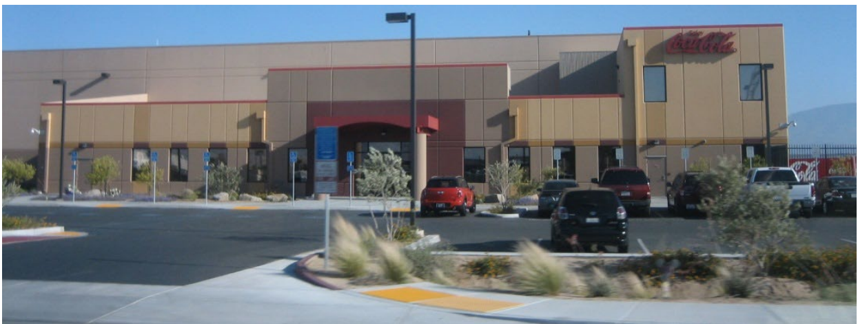
Large industrial manufacturing facility provides head of household jobs but should be distant from residential districts.
